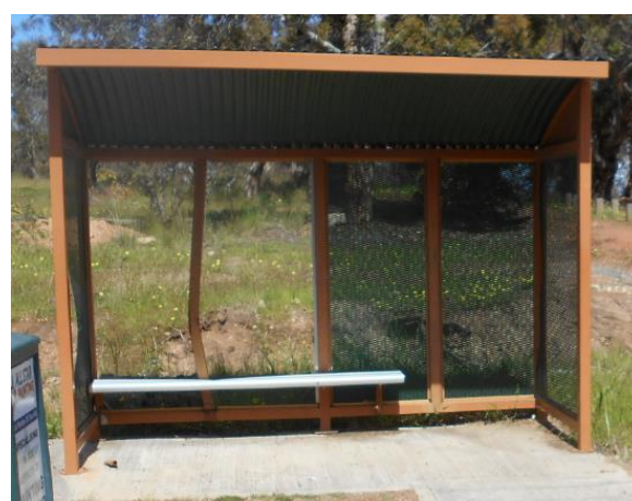
Steel bus shelter (Miricale) with vandalised panels
