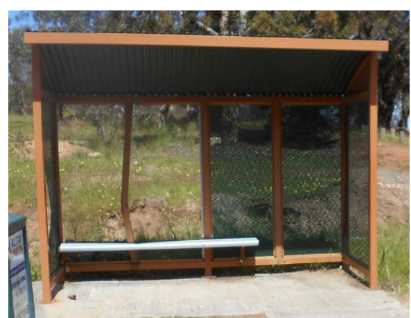
Steel bus shelter (Miricale) with vandalised panels
