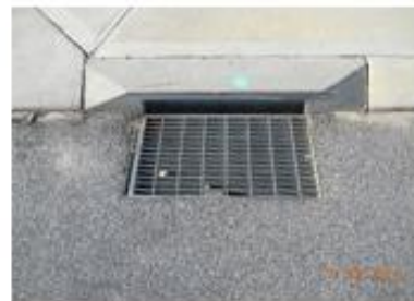
Side Entry Pits (left to right - single, double and grated)
