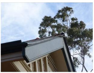
Figure 26 Damaged timberwork to gable end
