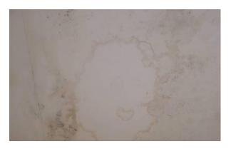
Figure 101 Water staining to ceiling of kitchen
