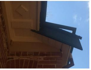
Figure 14 Exposed downpipe in gutter
