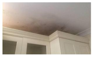
Figure 102 Water staining to ceiling of kitchen
