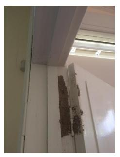
Figure 128 Sunroom, termite damage
