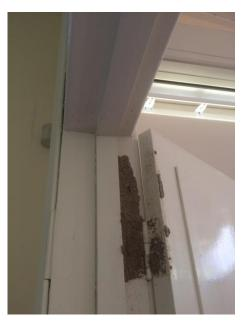
Figure 128 Sunroom, termite damage
