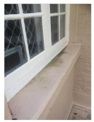
Figure 43 pressed metal capping to sill
