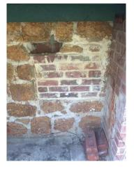
Figure 35 brick patch to wall behind condenser units
