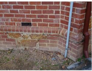
Figure 24 Fretted & damaged brickwork
