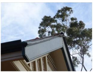
Figure 26 Damaged timberwork to gable end
