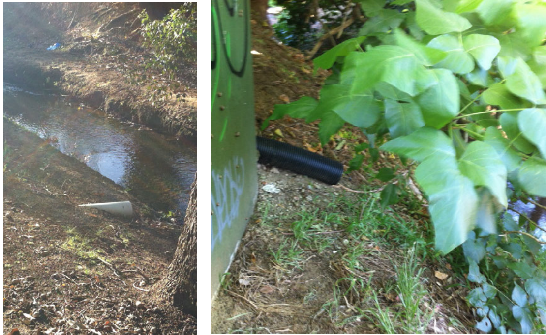
Plate 20: Minor local drainage discharges should discharge via vegetated overland flow
