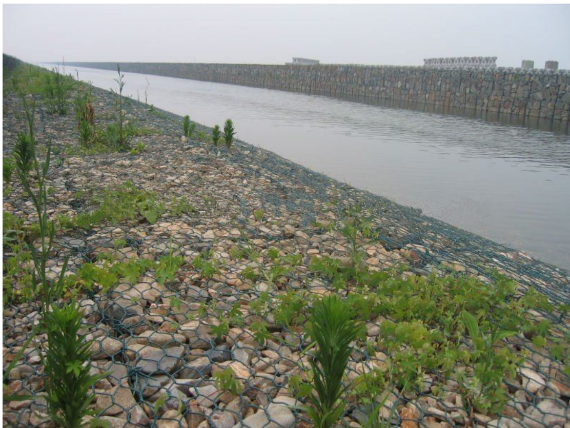
Plate 19: Example of vegetation growing within gabion walling
