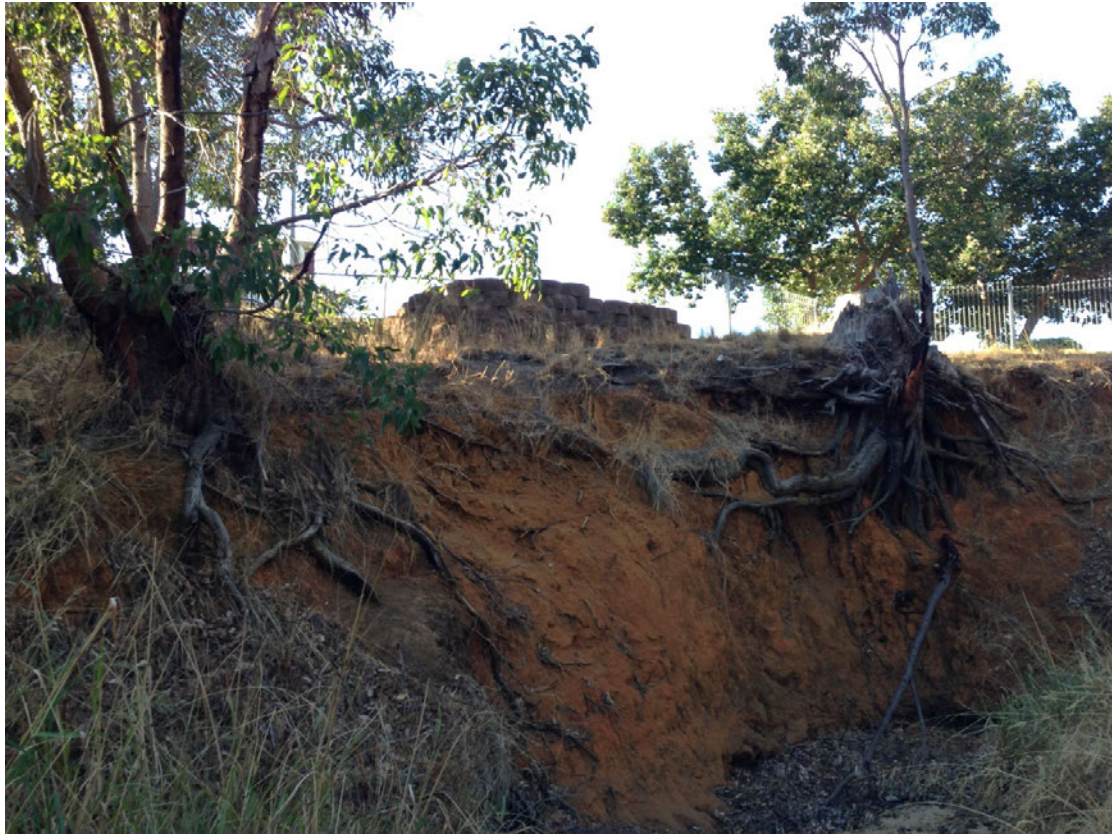
Plate 18: Severe erosion of bank undermining trees and threatening car park beyond
