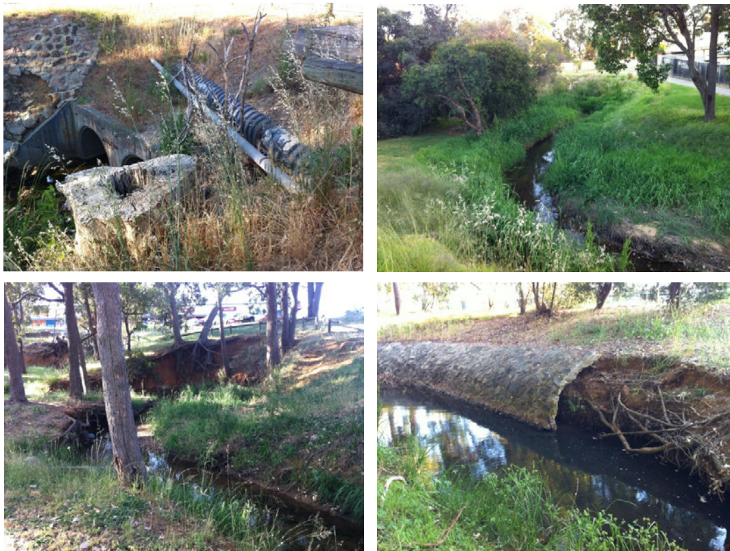
Plate 3: Evidence of weeds and undercut trees and reinforcements on Woodlupine Creek
