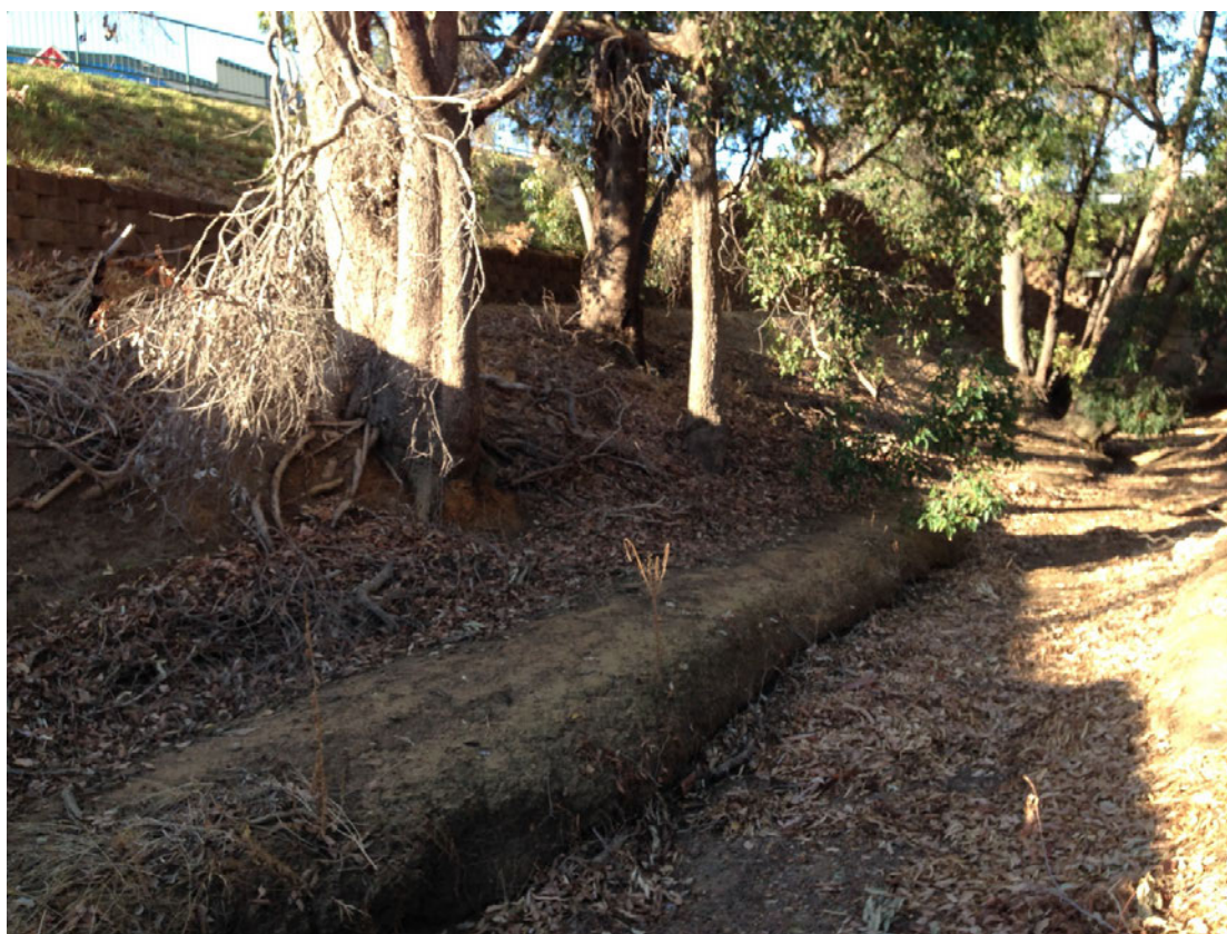
Plate 17: Erosion of bank at risk of undermining trees, retaining wall and car park beyond
