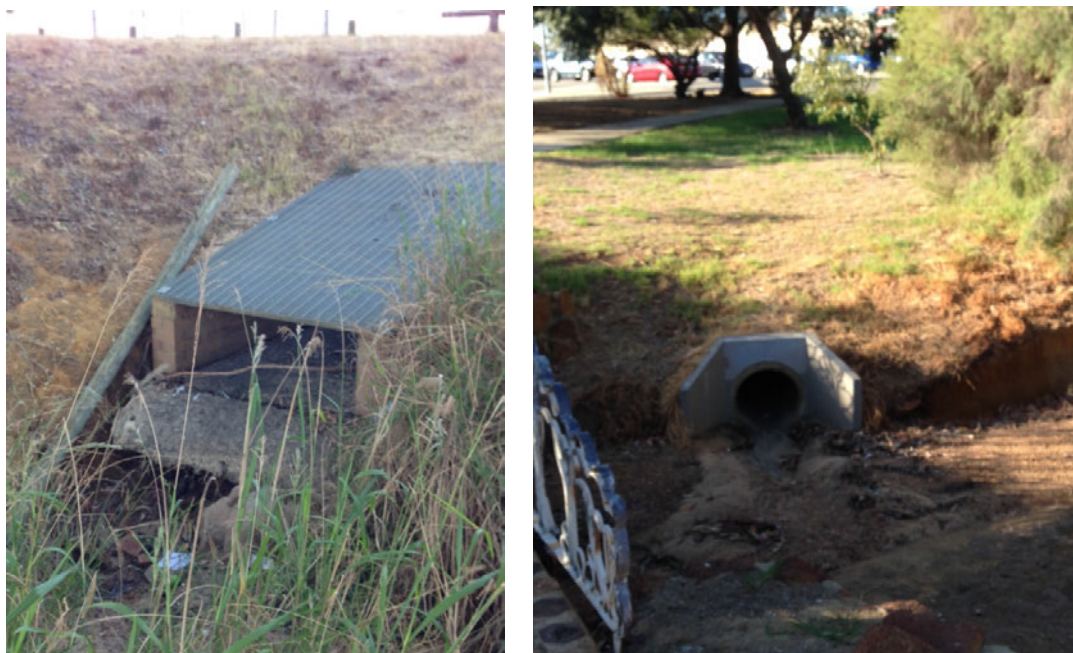
Plate 21: Local drainage discharge outlets requiring modification to limit erosion effects
