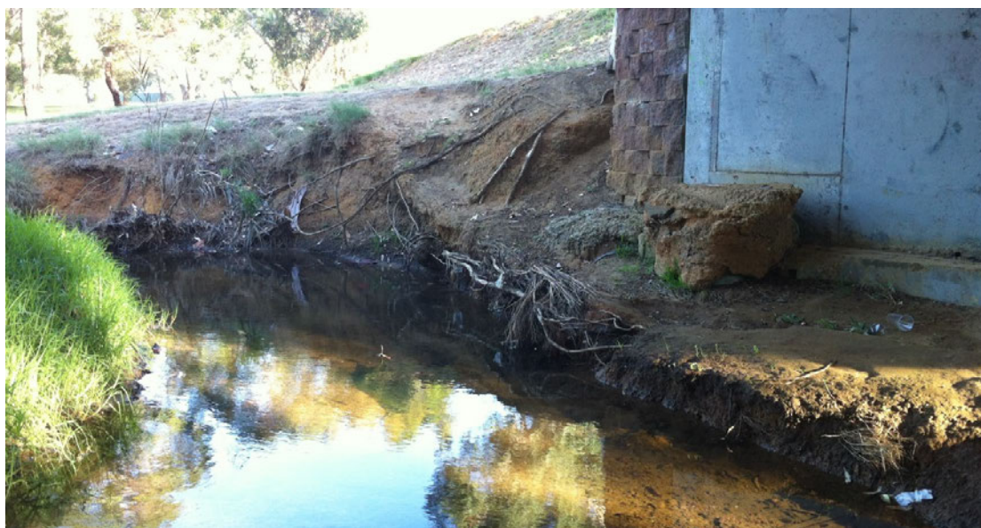
Plate 14: Existing structure requires protection from permeable stabilisation techniques
