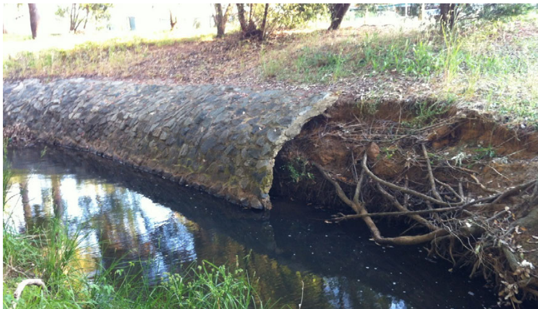
Plate 13: Existing structural stabilisation to be removed, bank behind requires bank slope reduction and revegetation or use of permeable stabilisation techniques.
