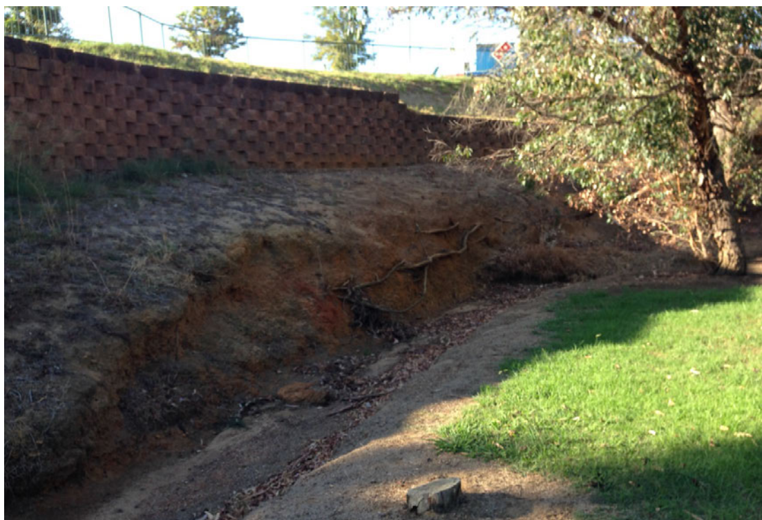
Plate 16: Erosion of outer bank at risk of undermining existing retaining wall, revegetation and bank stabilisation will be necessary to prevent further erosion
