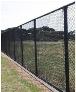
Fence, with flush 150mm concrete strip beneath
