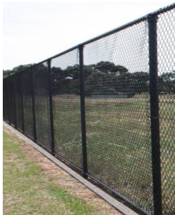
Fence with flush 150mm concrete strip beneath
