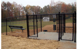
Double entry gates spring loaded
