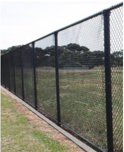
Fence with flush 150mm concrete strip beneath
