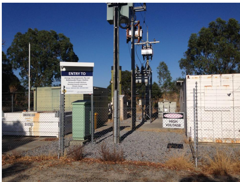
Figure 5-6: Grid connection for existing landfill-gas generator
