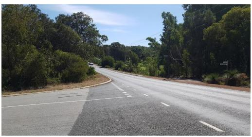
Photo 36: Visibility to the north is limited by both geometry and roadside vegetation.
