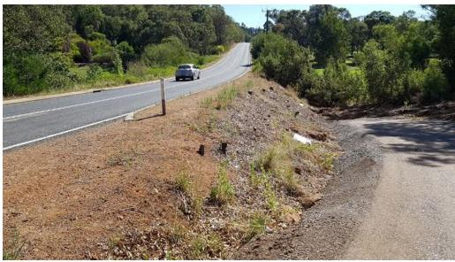
Photo 35: Unrecoverable batter with a significant drop off.
