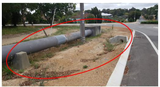
Photo 31: Pipe, concrete blocks, post and headwall – all remain exposed.
