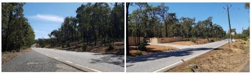
Photos 40 & 40a: Northern service road intersection joins Canning Road at an acute angle of around 20°.
