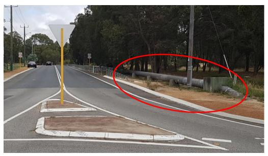
Photo 30: Wire rope safety fence does not cover these items.
