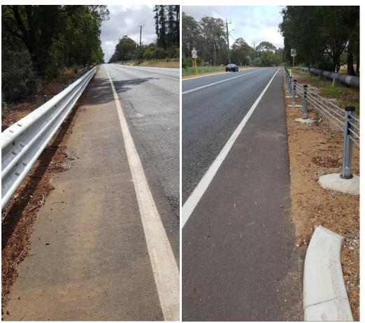
Photos 22 & 22a: Sealed shoulders are of sufficient width for cyclists to use, but are not to cycle lane standard.
