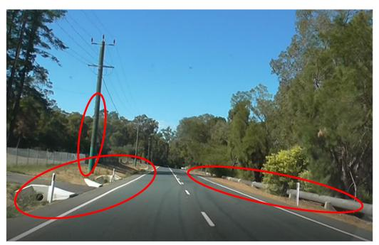
Photo 32: Concrete headwalls, piping and concrete blocks all provide hazards to errant vehicles.
