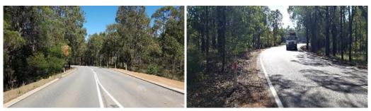
Photos 3 & 3a: The bend south of Pickering Brook Road is too sharp for the posted 70 km/h speed limit
