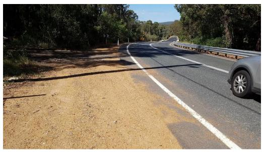
Photo 34: Loose material on hard shoulder and road surface.
