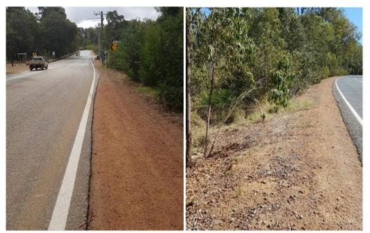
Photo 23 & 23a: The sealed shoulders along this section of Canning Road are almost negligible.
