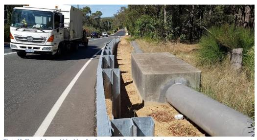
Photo 33: If struck by a vehicle, this safety fence may deflect further than the concrete block.
