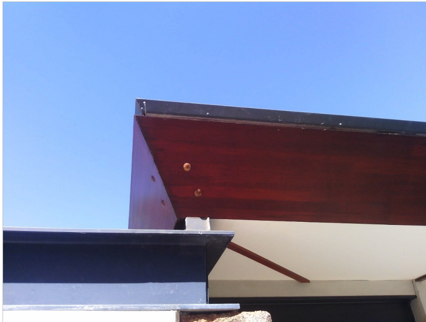
Renewal of roof flashing
