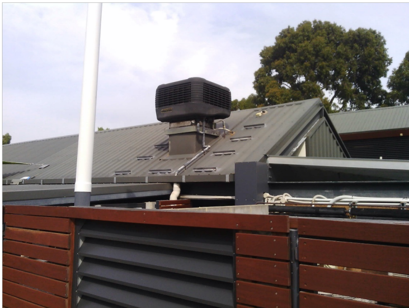
Replacement of evaporative air conditioners
