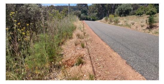
The third image shows typical treatment to back of open drain only. This prevents vegetation encroachment from damaging road surface and impeding the function of the drain.
