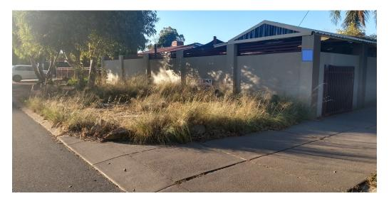
This picture shows that the verge has been covered with gravel and has soil piled up. This treatment is dangerous to mow, with projectiles from mower blades common. Mowing equipment is also often damaged, expensive to repair and not available to use whilst being repaired.
