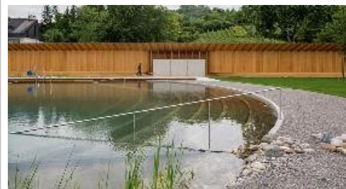
Riehen, Switzerland An outdoor pool kept clean using water plants as well as layers of gravel, sand and soil, rather than with machinery and chemicals.
