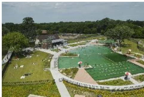
Riehen, Switzerland An outdoor pool kept clean using water plants as well as layers of gravel, sand and soil, rather than with machinery and chemicals.
