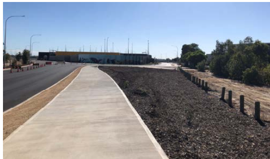
Figure 7-1 Maida Vale Road Intersection
