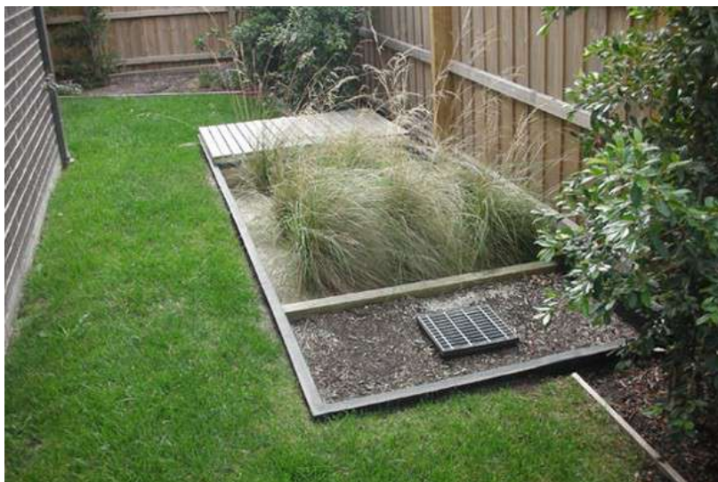
Plate 1: Lot scale bioretention systems
