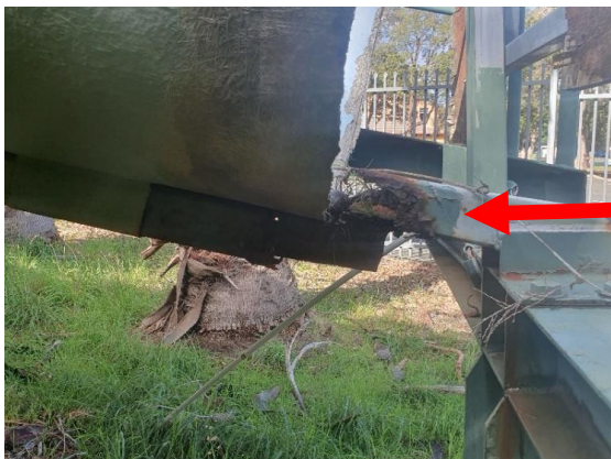
Figure 3 - Condition/Gap at end of Speed Slide
