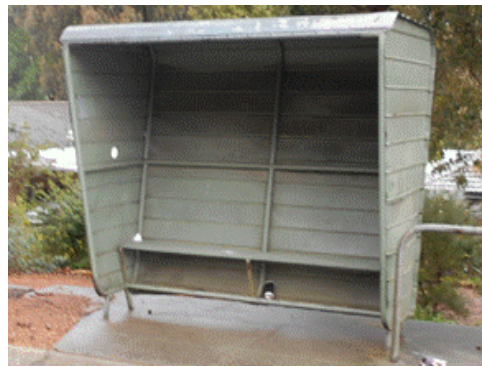
Typical tin bus shelter
