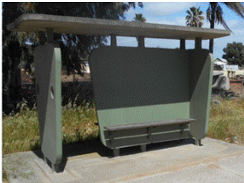
Typical concrete bus shelter
