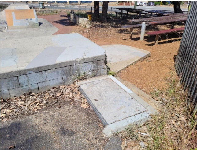
Figure 9-21: Storm Water Pits
