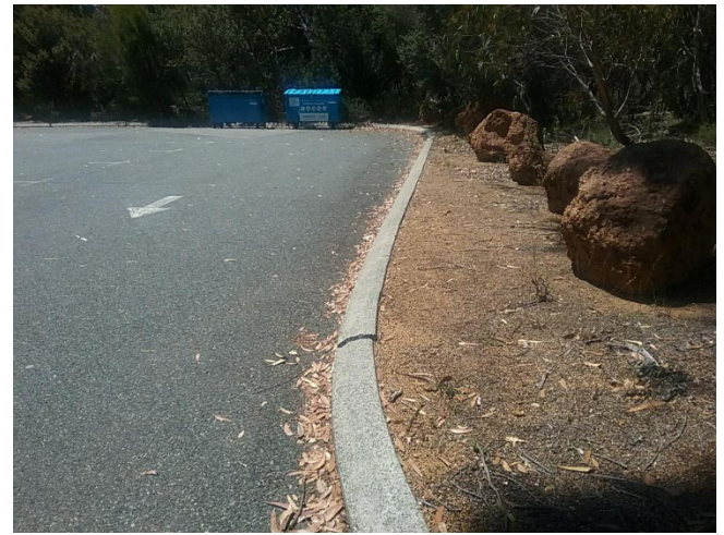
Figure 9-2: Kerb of Car Park 2
