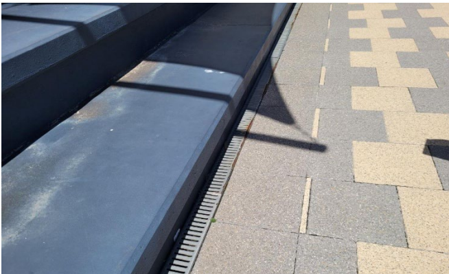
Figure 9-22: Surface drainage near the main pool
