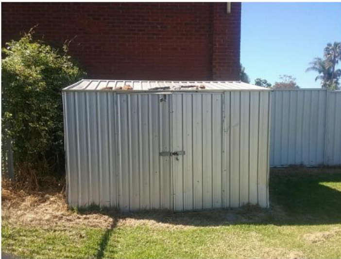
Figure 9-16: Storage shed behind the Rollerama
