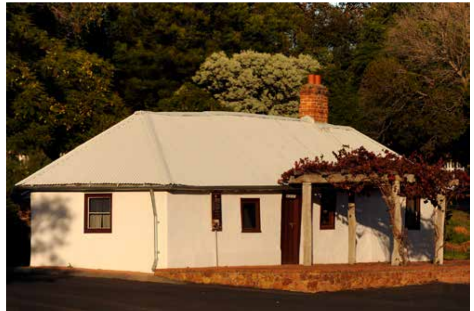
Figure 2. Stirk Cottage, supplied by the Shire of Kalamunda
