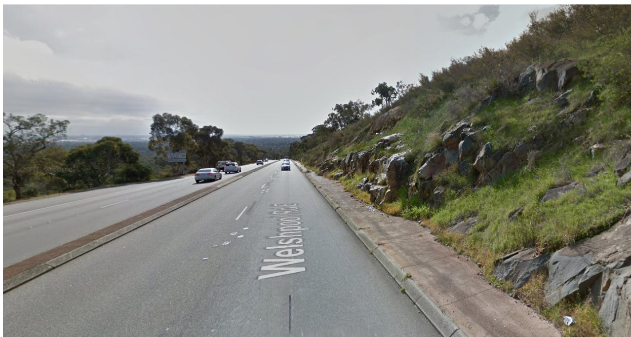
Photograph 4 – Challenging terrain on Welshpool Road East at Lesmurdie Hill
