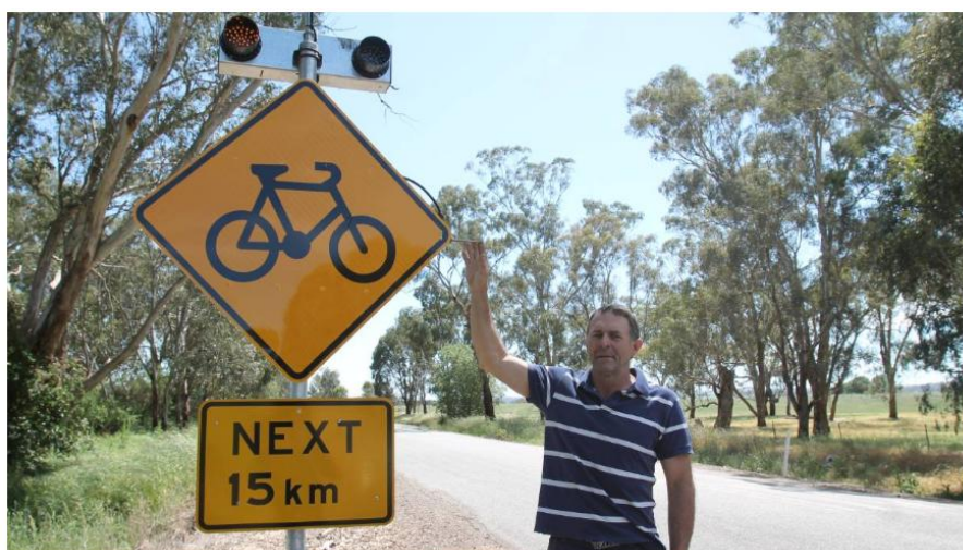
Figure 7-28 Examples of activated warning sign – Cootamundra NSW
