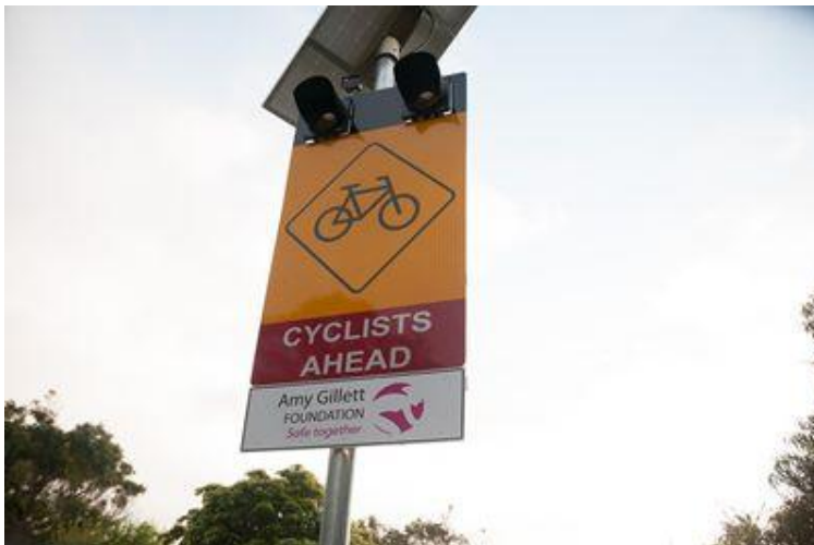
Figure 7-27 Examples of activated warning sign – Victoria
