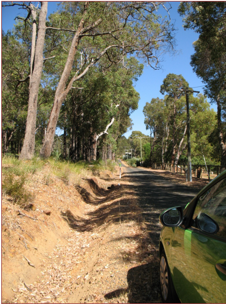
Plate 3-2: Road drainage on Marchetti Road
