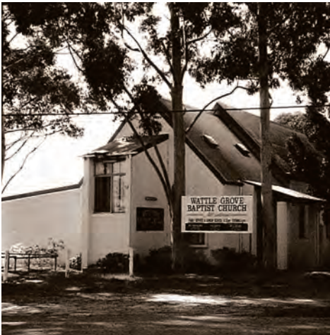
The Wattle Grove Baptist Church.
