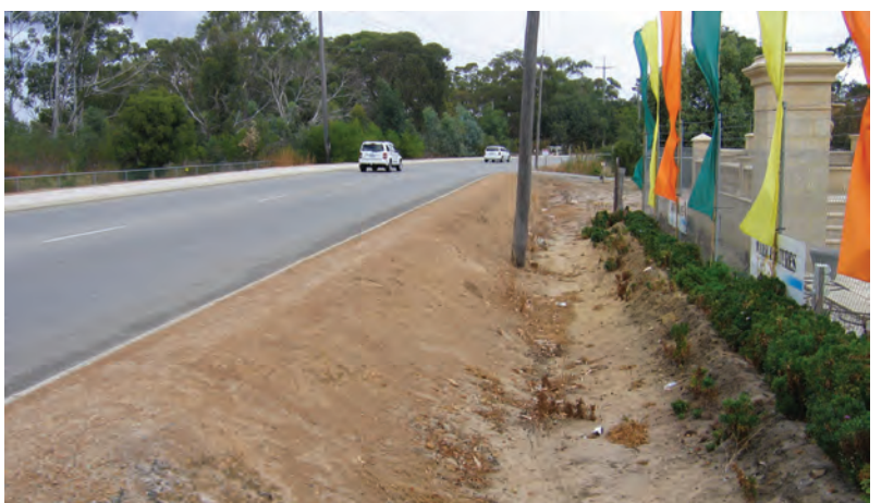
Hale Road is bordered by spoon drains and overhead power lines.
