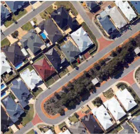
Designers of the Harvest Edge development identified existing trees for retention and accommodated them in the road design; creating a loop and 'mini' park which also filters storm water.
