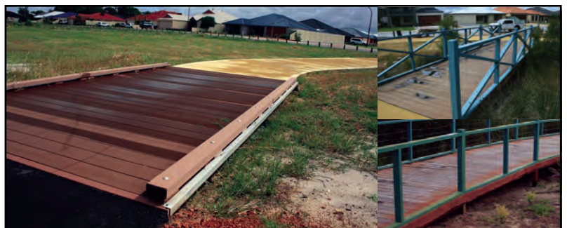
DECK/BRIDGE: BY LANDMARK, TIMARU TIMBER BOARDWALK WITH EINWOOD DECKING
