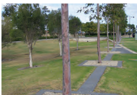
This grassed swale at Heron Park helps manage storm water.
