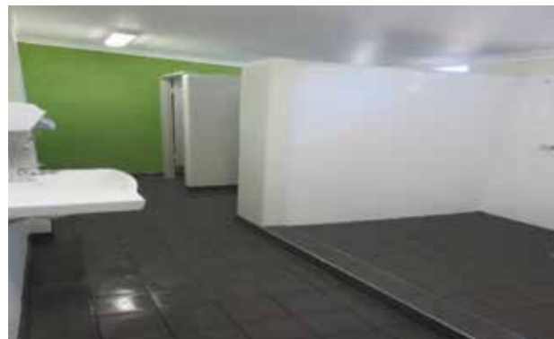
Completed Toilet Refurbishment
