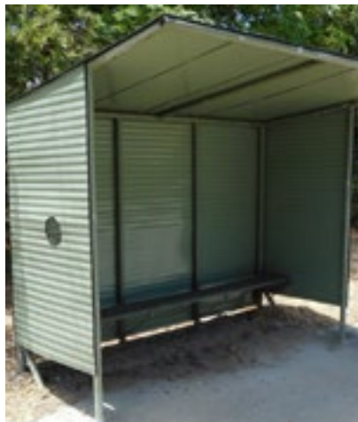
Bus Shelter - after
