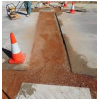
Berberis Way drainage upgrade
