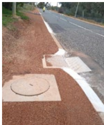
Holmes Road drainage upgrade
