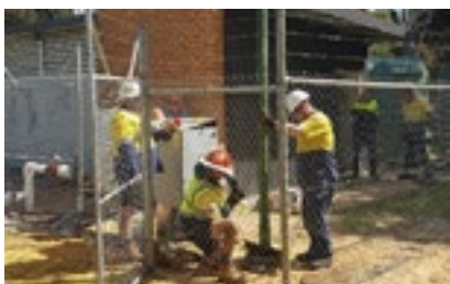
Carbon filters and injection pipework being installed at the MAR
