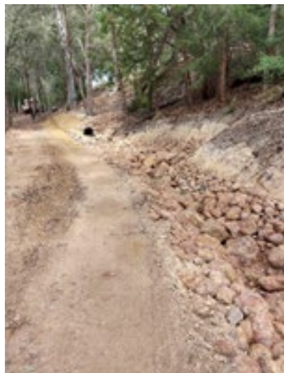
Firebreak drainage upgrades - John Street, Gooseberry Hill
