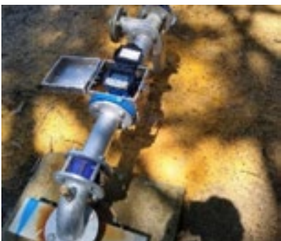
Upgrade of the Bore headworks with a New Octave ultrasonic water meter fitted at the MAR
