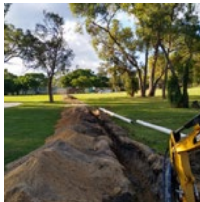
Rangeview Reserve playground upgrade
