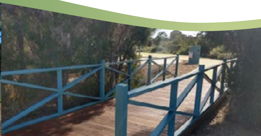
Maamba Road Reserve Footbridge
