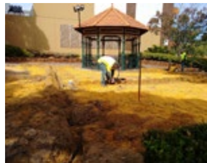
Town Square reticulation install
