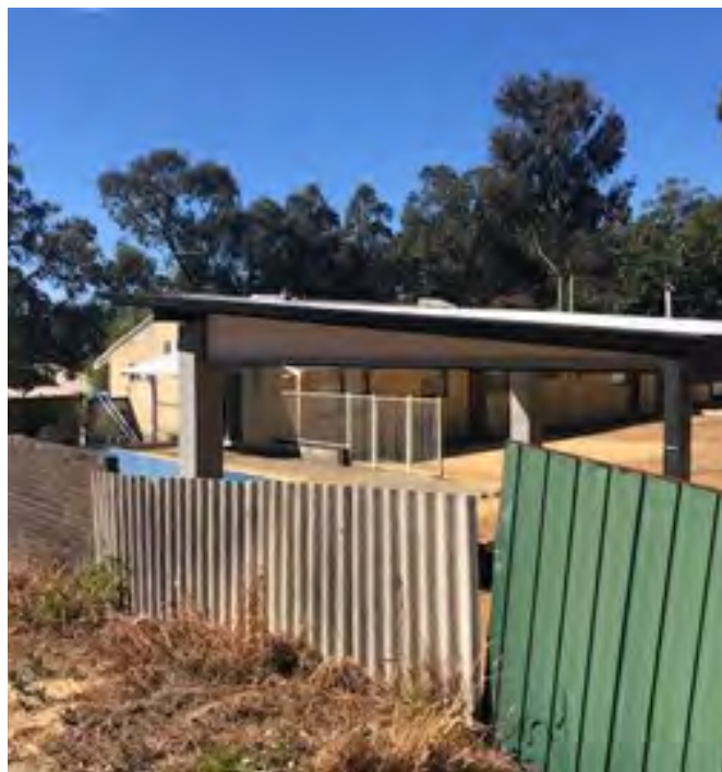
Example of non-compliant Swimming Pool
