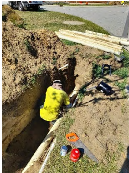
City Reticulation repairer repairing a pipe at Gala Way Reserve
