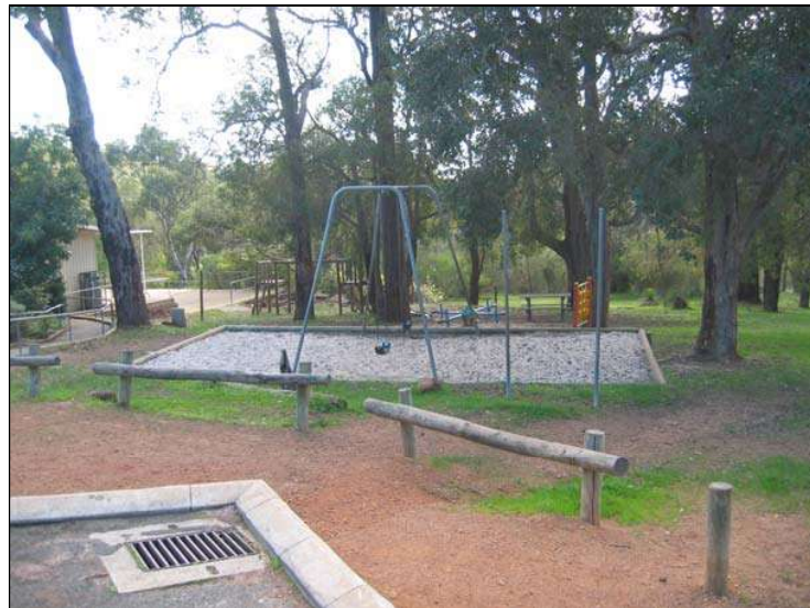
Figure 21: Loose gravel and eroded areas at access point
