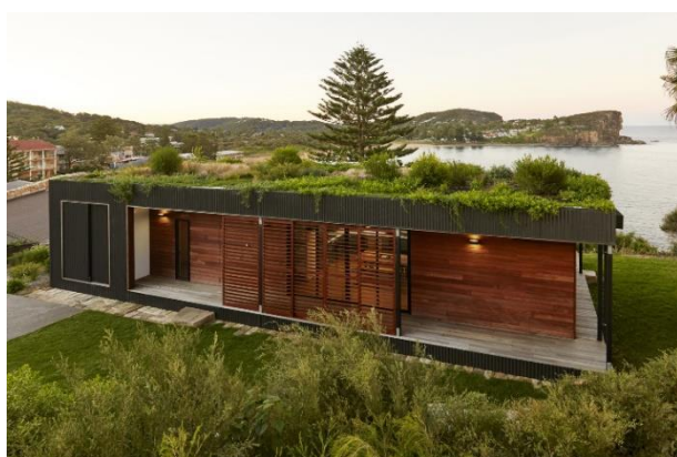
Figure 40. Example of a modular home (Source: Archiblox. 2019)
