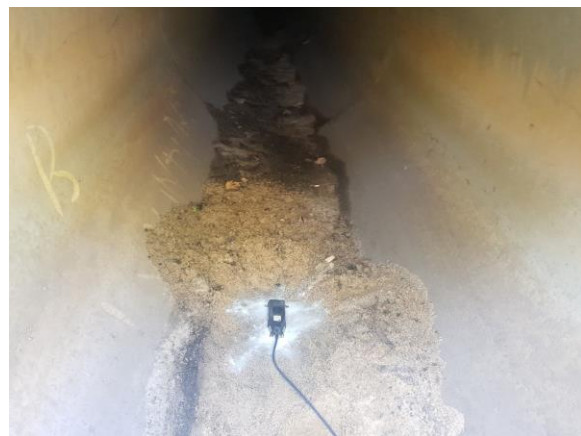
Doppler Sensor installed at Crumpet Creek
