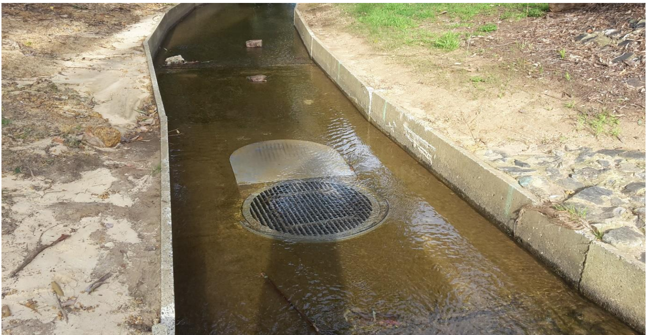
Woodlupine Main Drain stormwater extraction point
