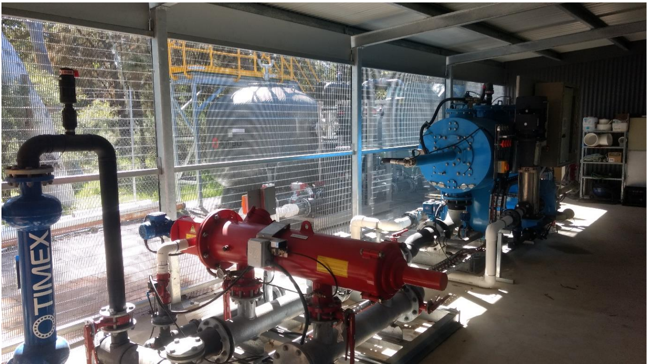
Hartfield Park MAR Filter System
