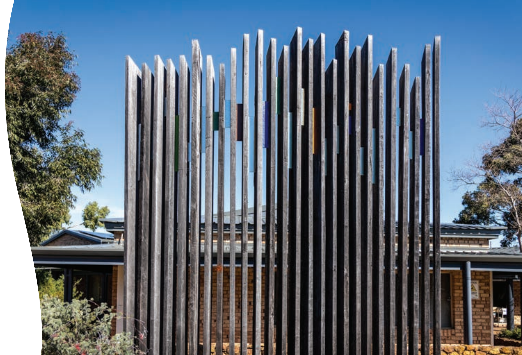
3. Scarp 1 and Scarp 2, 2011, front of Library to Williams St and Railway Rd
